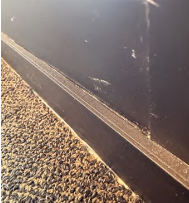
Photo #1: Floor slab is visible between carpet and window sill.
