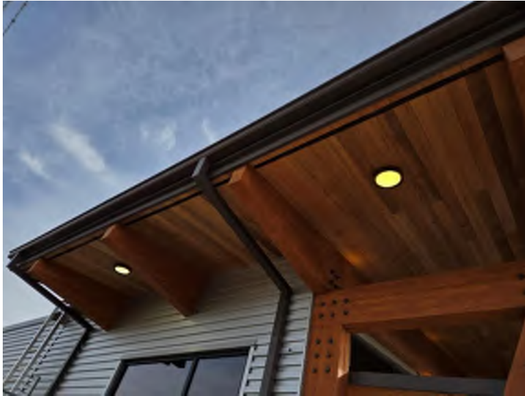
Exterior Fixtures Appear Different Color Temperature
