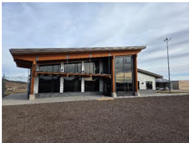
Exterior Air Side
