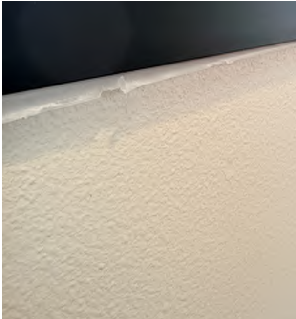
Photo #35: Floor sink requires caulking at perimeter. Also needs to be cleaned out.
