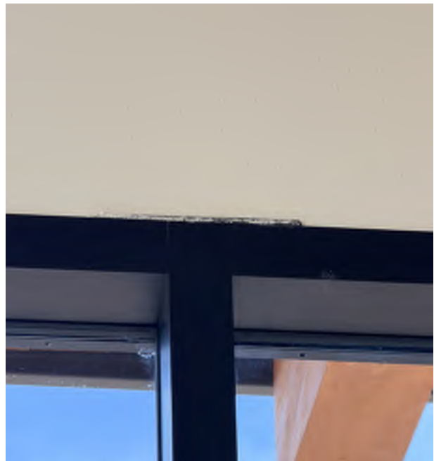
Photo #40: Connection plates visible above West curtain wall.
