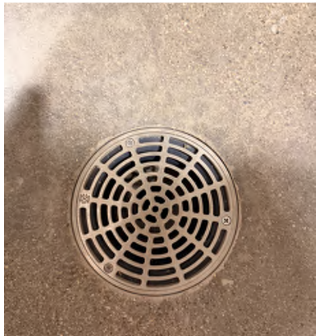
Photo #72: Provide sealant around floor drain assembly. Typical at all locations.
