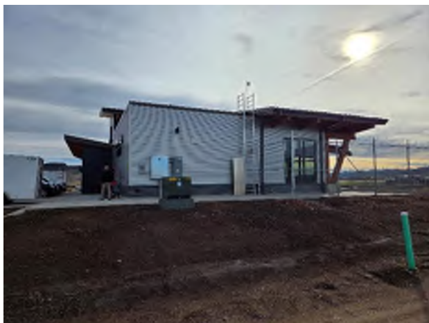
Exterior West Side
