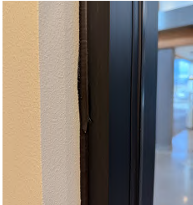
Photo #24: Messy caulk at window in Flight Planning 105
