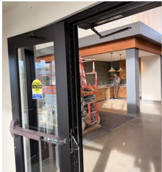
Photo #32: Finish door hardware install for Door 110C
