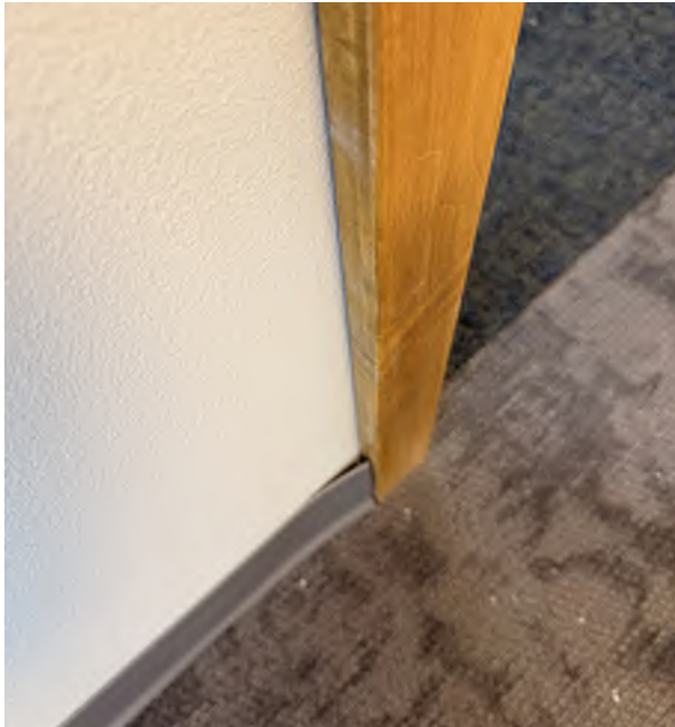
Photo #27: Finish door casing installation. Trim and adhere wall base as required.
