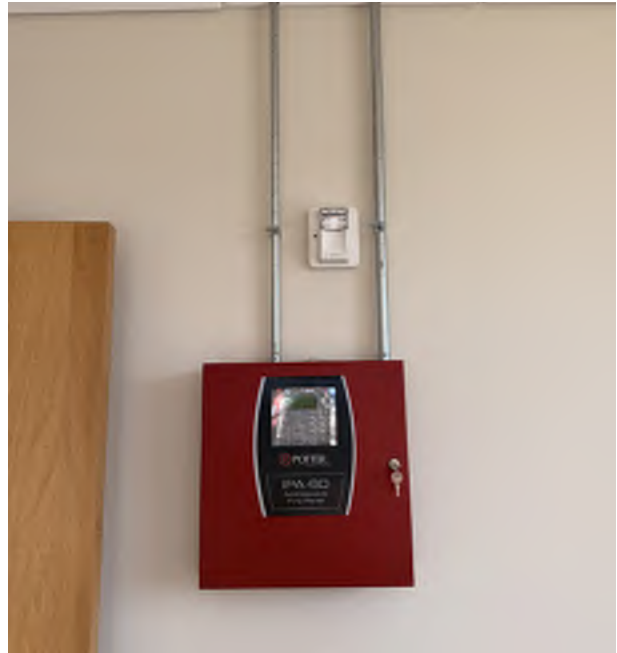
Photo #28: Paint exposed conduit to match wall behind.
