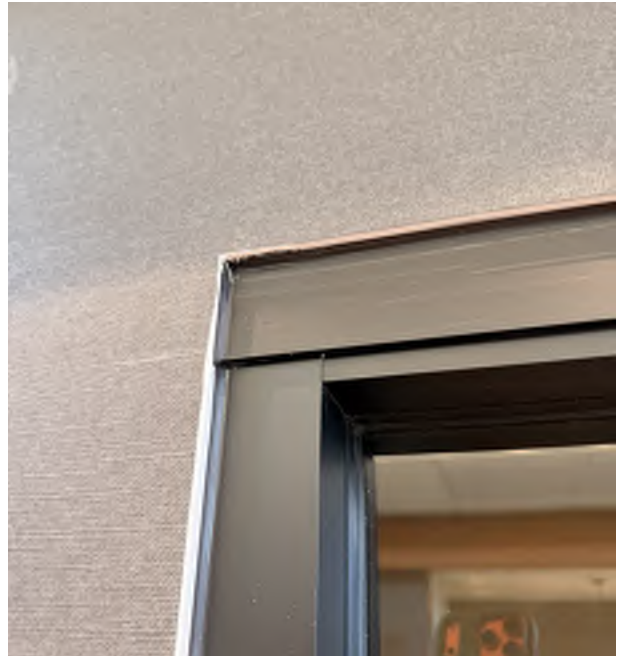
Photo #10: Wall covering fibers visible at head of window into Flight Planning 105
